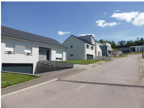
Figure 58 : Descente de garage
